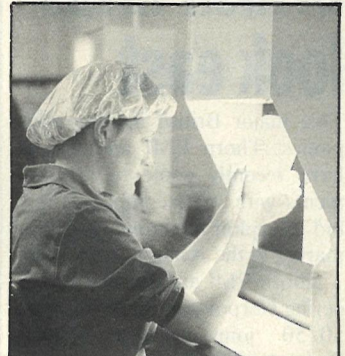
Inspecting sterile fluid in the laboratory with an illuminated viewer (West Midlands Regional Health Authority.)
